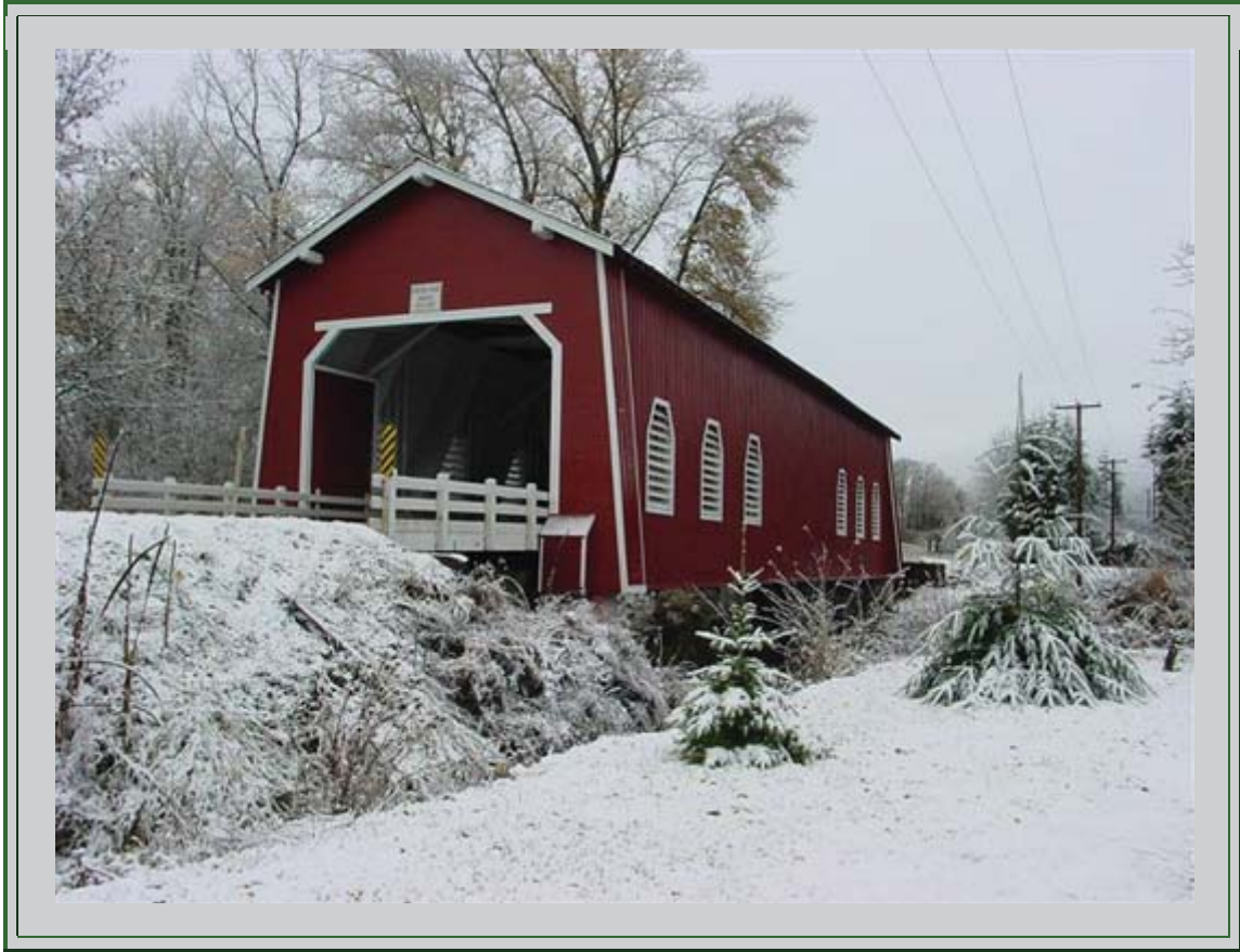
Shimanek Bridge - Photo by: Tom Rogers
