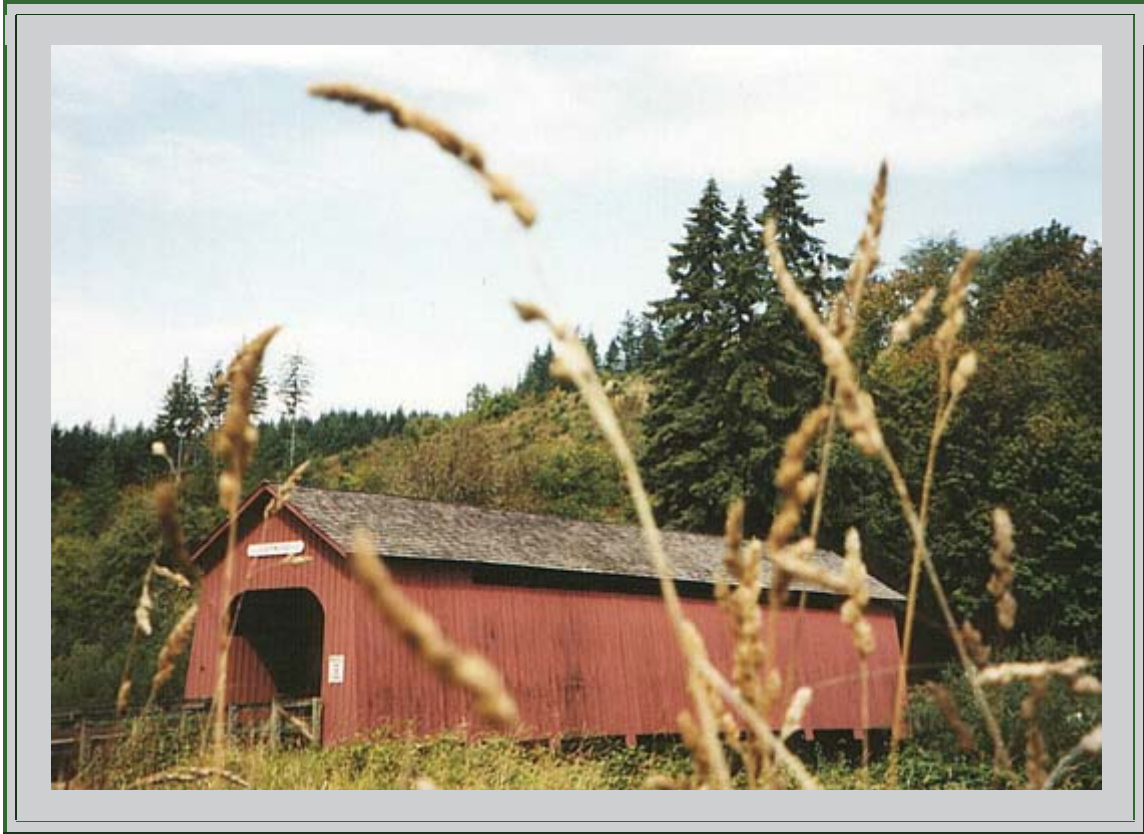
Chitwood Bridge - Photo by: Judy Prindel
