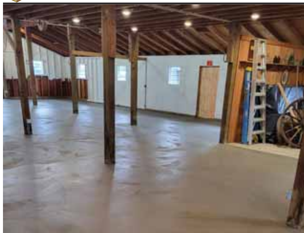
Above: The new concrete floor looks great in the farm museum.
