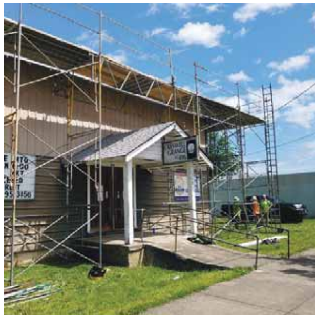
The scaffolding at the front of the hall.
