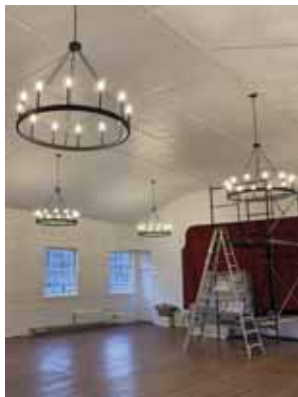
Above: Scaffolding was needed to paint, patch and apply the furring strips to the ceiling.
