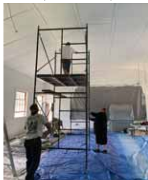
Above: Scaffolding was needed to paint, patch and apply the furring strips to the ceiling.
