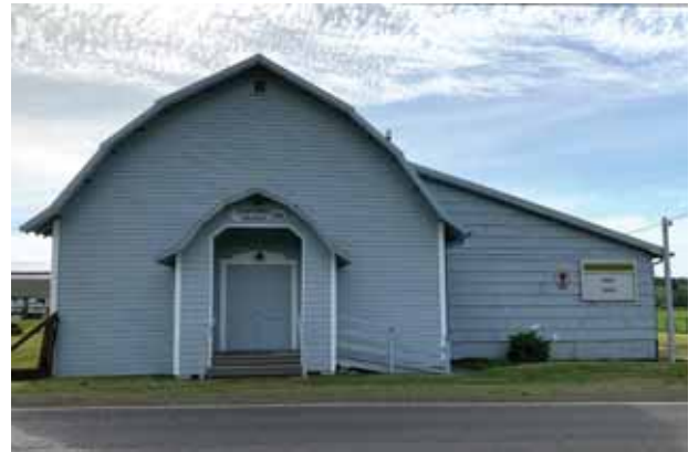
Sandlake Grange has a new reader board thanks in part to the Oregon State Grange Sign Reimbursement program.
