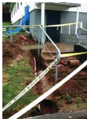
wet, cold, dirty job.
