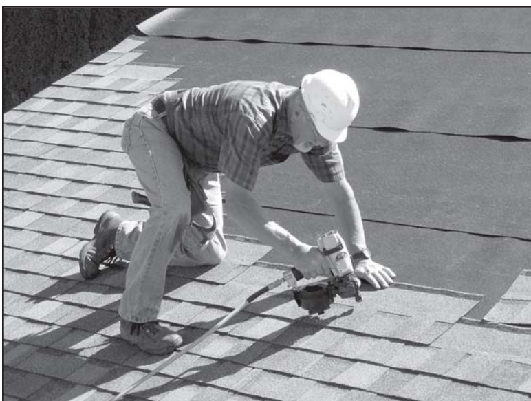
Gary Bush installs roof shingles
