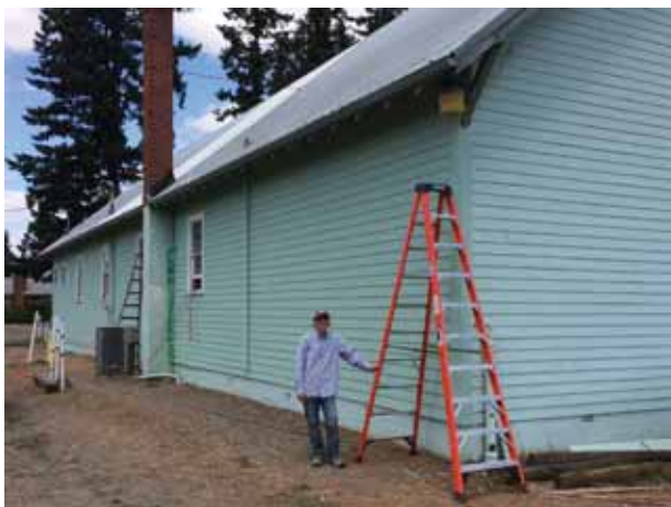
Above: the old bubbling siding was removed from the Grange hall and replaced with Hardiplank siding. Below: what a difference it makes.
